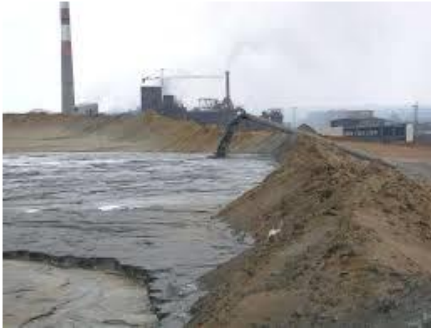
Figure 2. 1. Deposition of BCL mine tailing into dam
