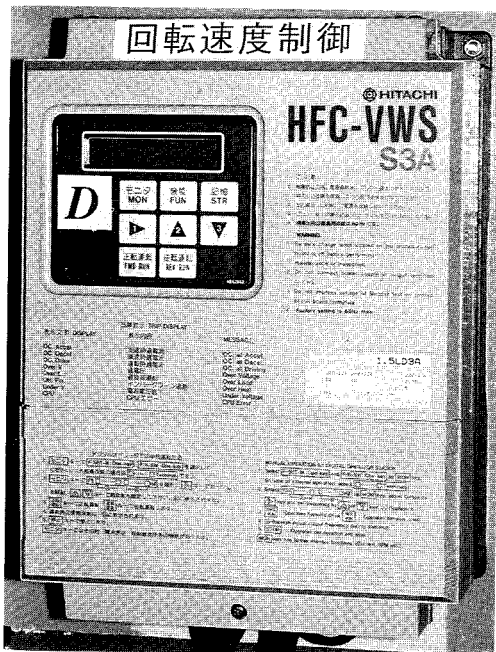
Fig. 3 Slurry speed control inverter.
